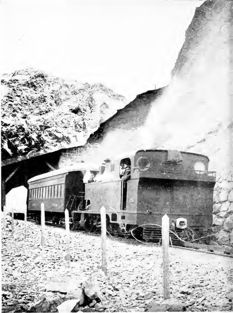
AVALANCHE SHED TRANS-ANDIAN RAILWAY
